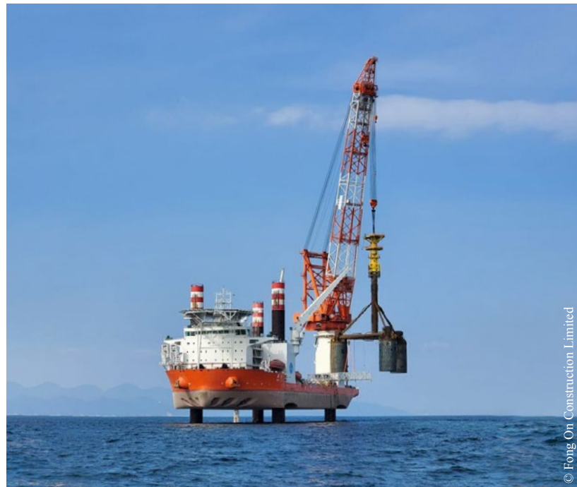
Arup was commissioned to design a wind mast to measure wind speed and other related data, using suction caisson foundations for the first time. This was to help CLP determine the viability of a larger-scale wind farm project.
