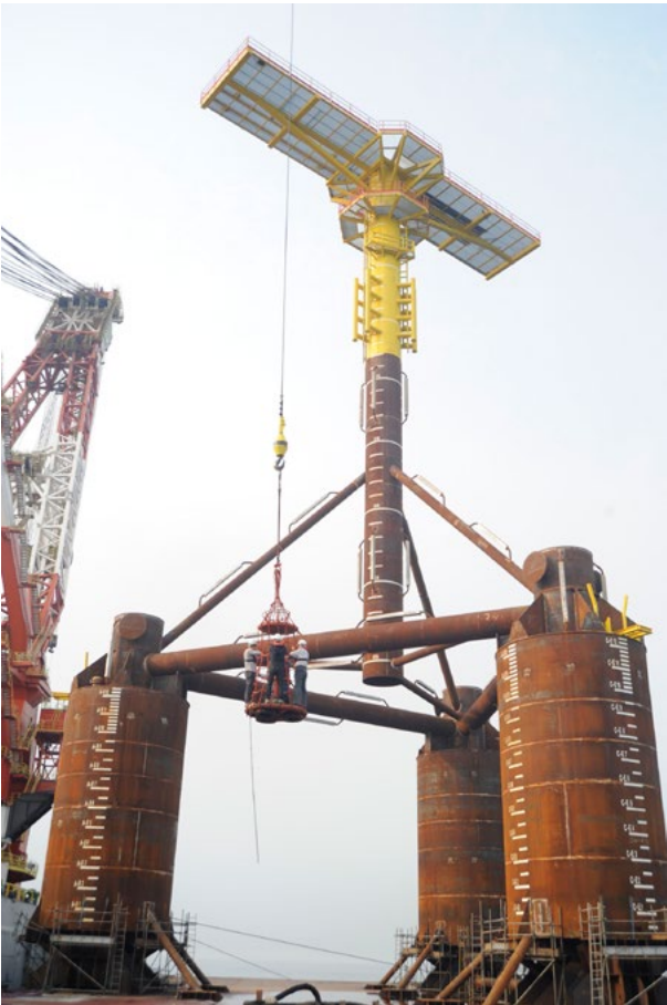
Arup pioneered the development for the design for the suction bucket jacket structure, performed site-specific and wind turbine generator-specific Integrated Loads Analysis for at least two wind turbine generator models.
